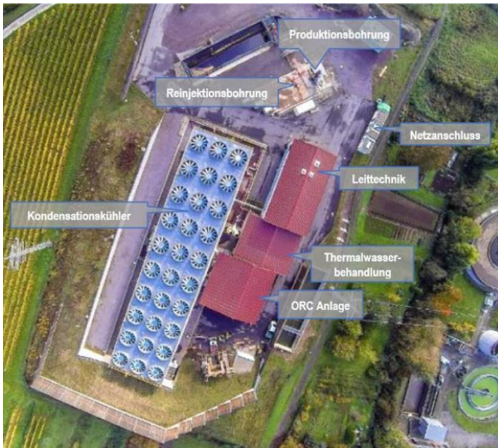
FIGURE 2-15 OVERVIEW OF THE INSHEIM GEOTHERMAL PLANT
