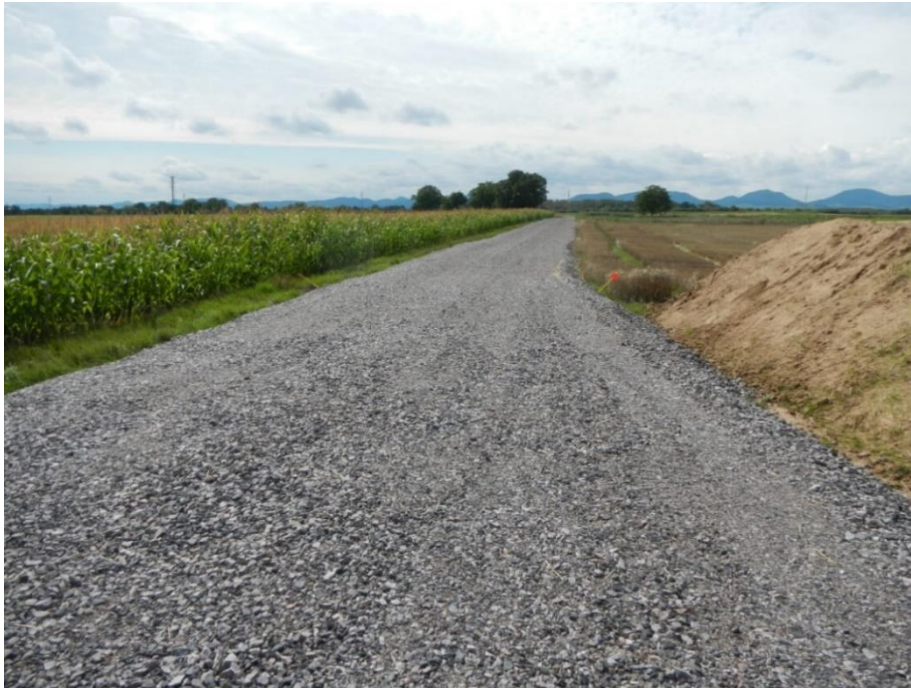
FIGURE 2-6 ACCESS ROAD FOR SCHLEIDBERG WELL SITE
