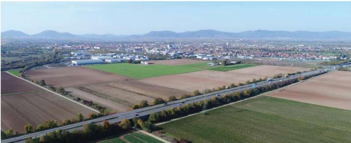
FIGURE 2-13 AERIAL OVERVIEW OF THE LAND PLOT FOR THE GEOTHERMAL AND LITHIUM PRODUCTION PLANT (GLEP)
