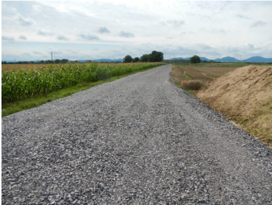
FIGURE 2-6 ACCESS ROAD FOR SCHLEIDBERG WELL SITE
