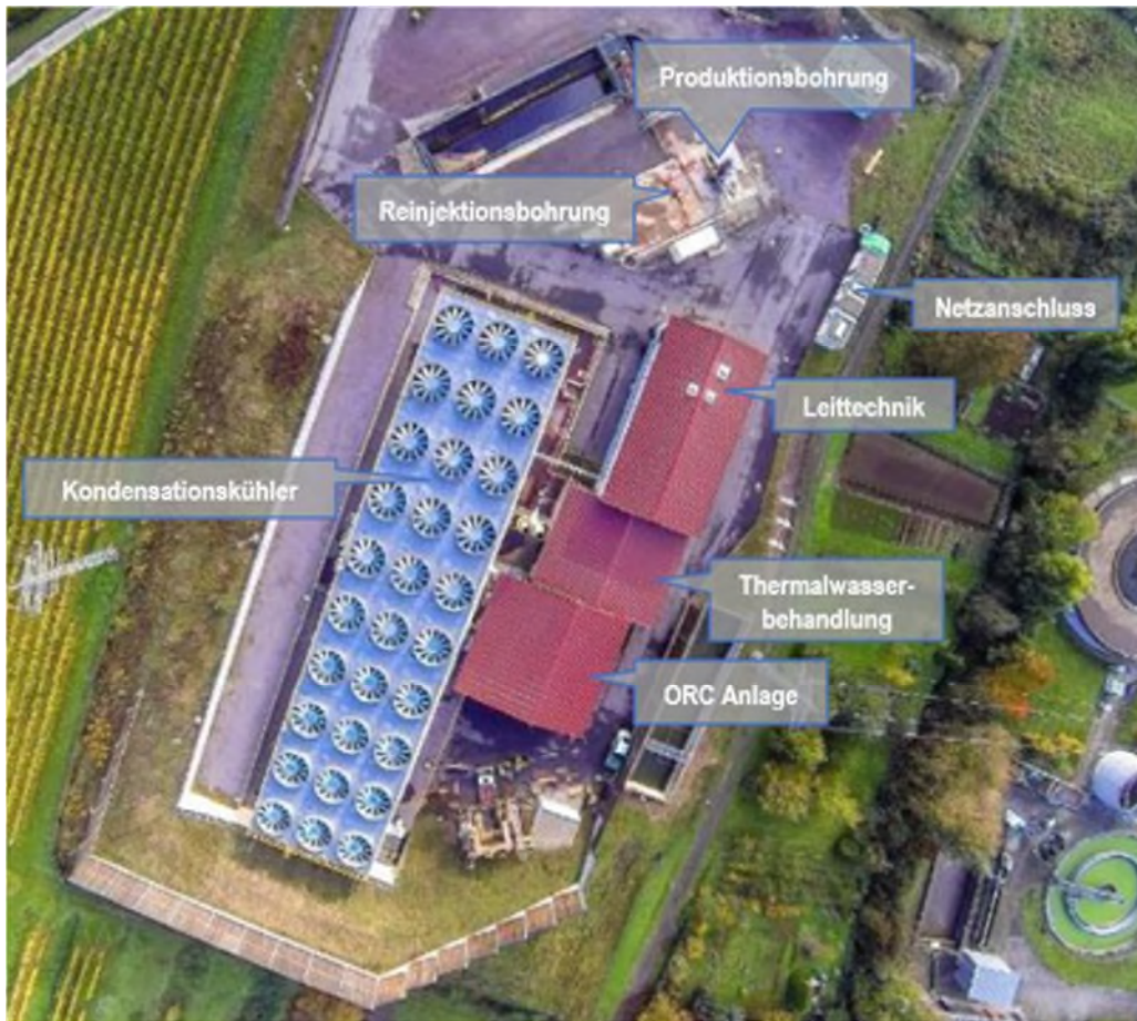
FIGURE 2-15 OVERVIEW OF THE INSHEIM GEOTHERMAL PLANT
